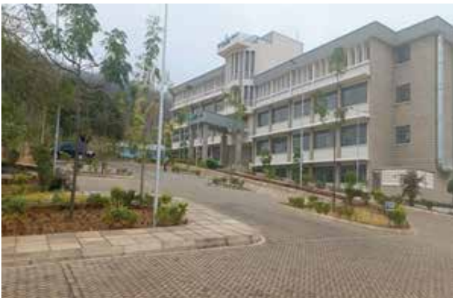
A front view of Wote Campus Office and Tuition Block
